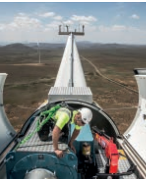
Construction at Loeriesfontein Wind Farm, South Africa.
