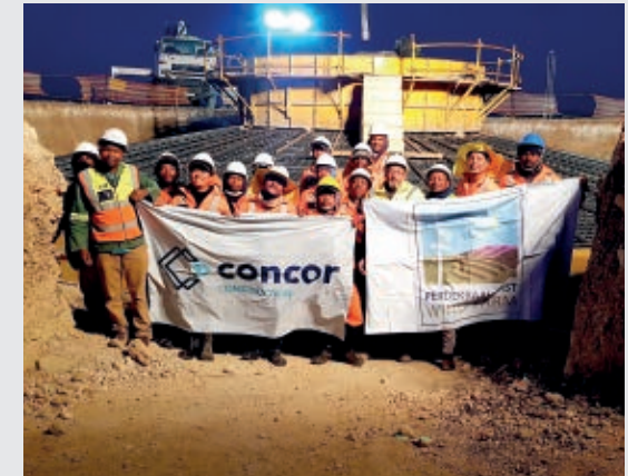
Construction at Perdekraal East wind farm using 70% replacement of cement
