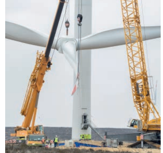
Construction at Sarco wind farm, Chile
